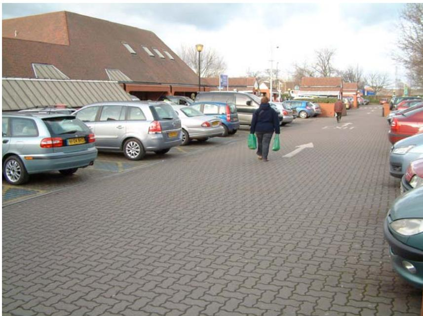
**Figure 6 Photograph (b) showing condition of supermarket block paving, constructed circa 1983**
