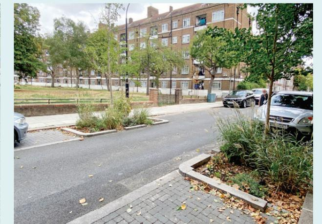
Two different profile examples of typical street enhancements in Hammersmith & Fulham, London (case study via [www.mpaprecast.org](http://www.mpaprecast.org)), characterised by low-intervention CBPP on-street parking. As well as delivering SuDS and irrigation for trees, the puddle-free CBPP retains litter, silt and pollutants on the surface for removal with straightforward cleaning.
