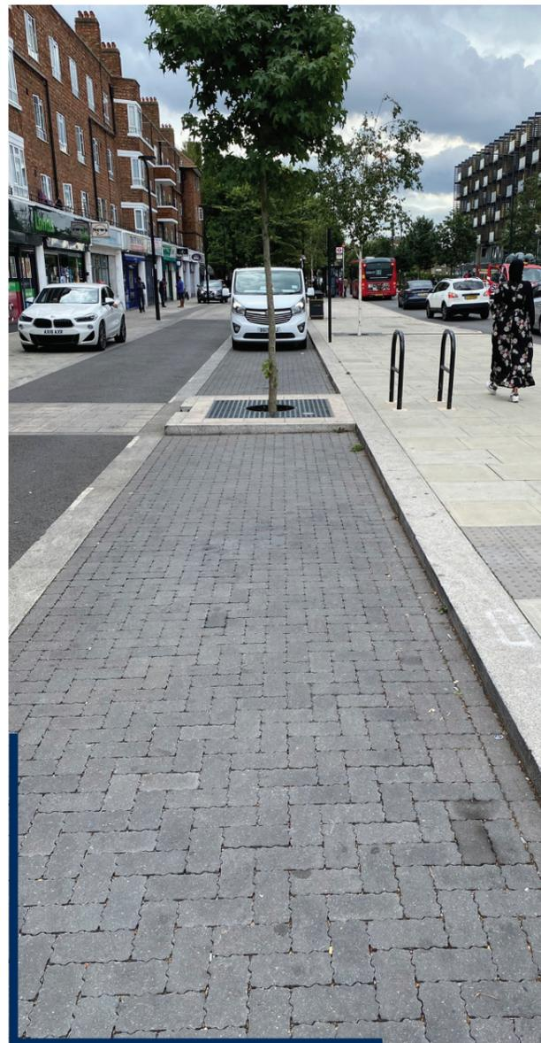
“CBPP works in synergy with trees, replicating natural permeable surfaces with diffuse rainwater infiltration and retention plus free air movement”.
