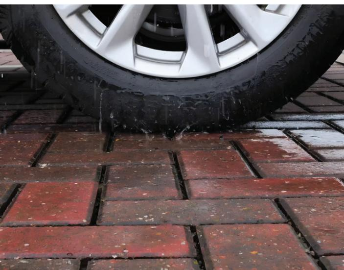
In contrast, rainwater drains straight off each block in CBPP, through the joints and laying course, as a permeable surface with dispersed drainage. CBPP attenuates and temporarily stores water during rainfall, cleaning, conveying and releasing it gradually over time. Essentially, it addresses flooding and water quality issues together, unlike attenuation tanks which only address flooding.
