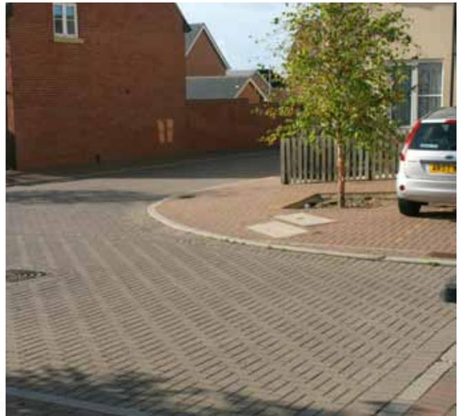
Concrete block permeable paving with conventional block-paved footways/ parking and flat kerb delineation.
