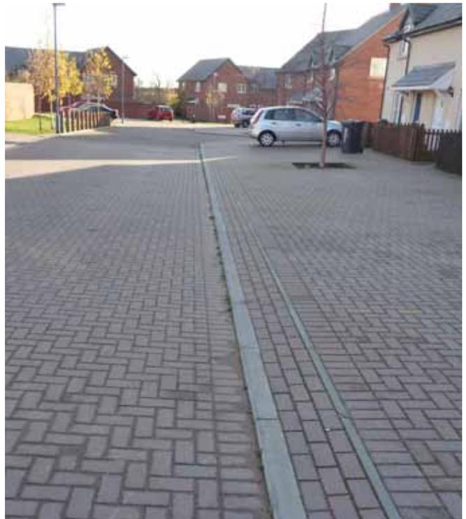
Precast concrete kerbs and various block laying patterns differentiate areas of paving.
