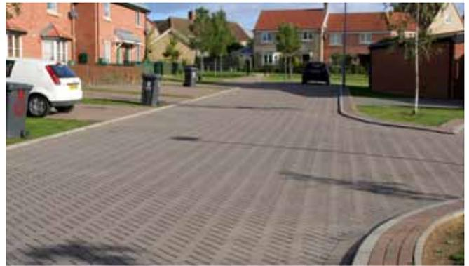
Concrete block permeable paved carriageway accepting runoff from conventional block paved drives and parking areas. Concrete kerbs laid flat delineate road edges.
