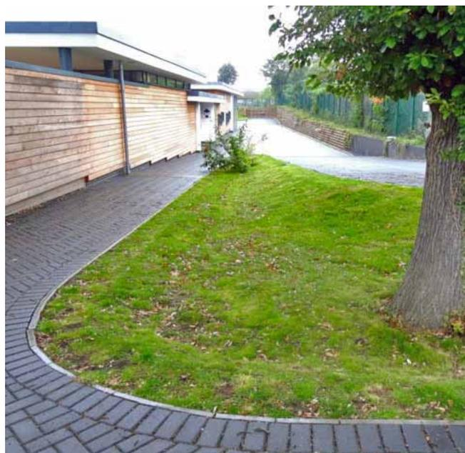
Permeable paving and a swale help irrigation of the mature oak tree.
