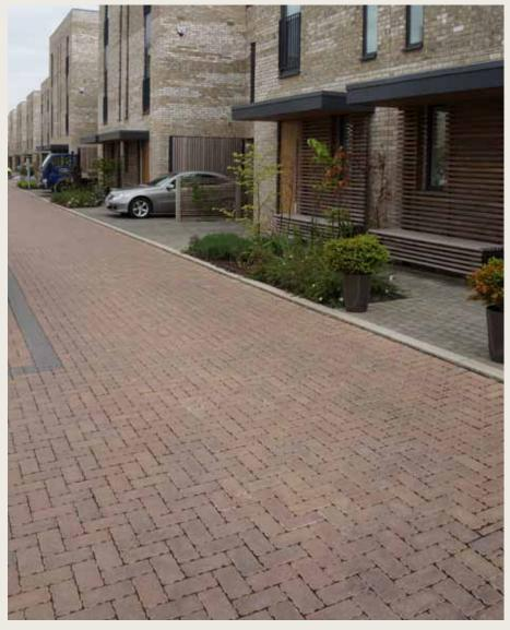
The division between public and private is signalled with enhanced finish concrete kerbs set flush, a change in block paving colour and planting, while retaining the openness of the main square.
