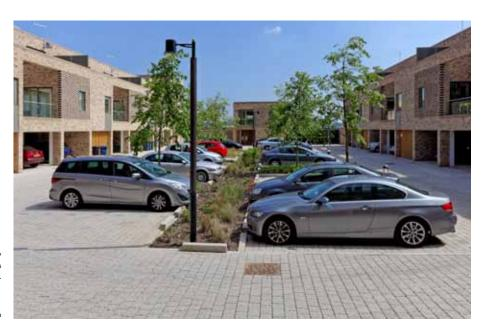
Concrete block permeable paving (foreground) infiltrates directly to the ground while matching conventional block paving drains between concrete kerbs onto a rain garden.
