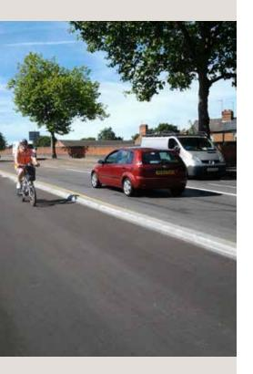
Following its role on London's CS2, the new precast concrete cycleway segregation kerb system is being used for a similar programme in Nottingham.
