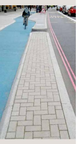
The new precast concrete cycleway segregation kerb units were first used on an upgrade to Cycle Superhighway 2 (CS2) between Bow and Aldgate.
