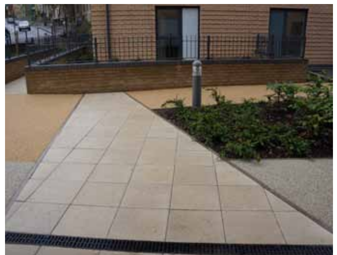
Enhanced finish concrete paving flags clearly identify the entrances to the Phase 1 blocks
