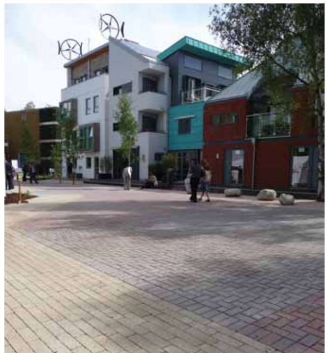
Concrete block permeable paving at the BRE Innovation Park
