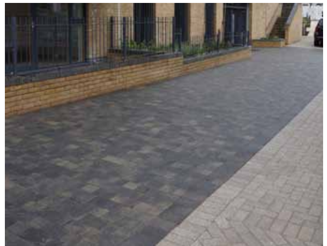
Light and dark concrete block paving defines vehicular and pedestrian areas behind Phase 1
