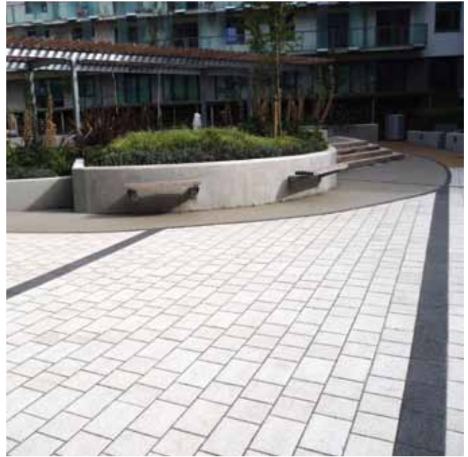
Granite finish concrete block paving at Forum House Wembley
