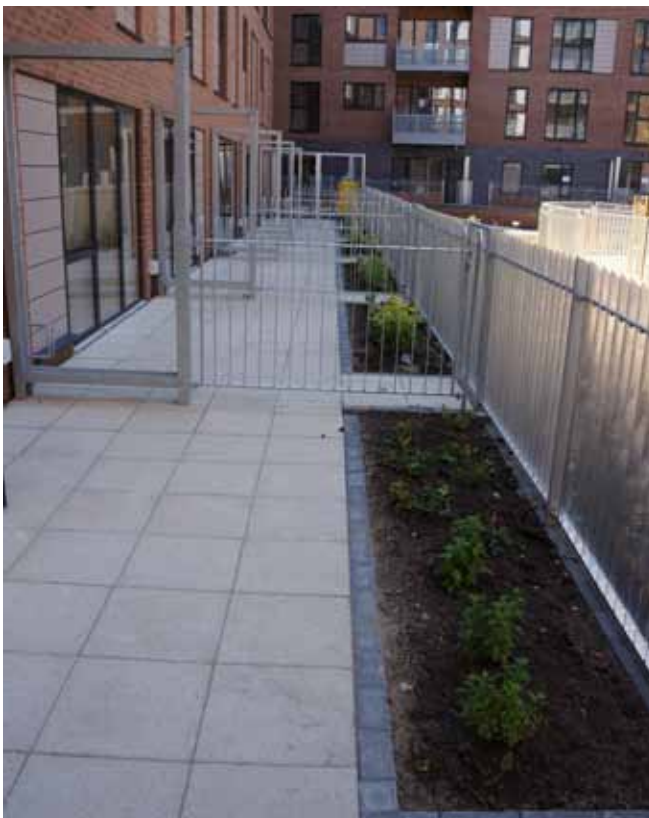
Private terraces surrounding the courtyard have precast concrete flag paving
