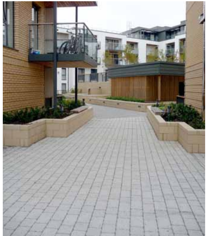
Concrete block permeable paving used for internal courtyards
