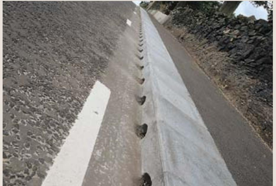
Precast concrete kerbs systems are available with integral drainage facilities
