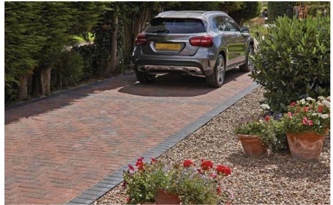
**Impermeable Surfaces** – such as conventional concrete block paving with sand joints, draining on-site to:
