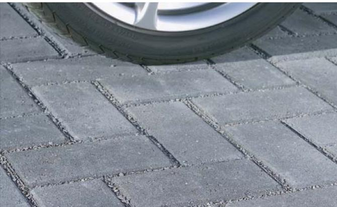
Permeable paving should have permeable aggregate filling the joints
