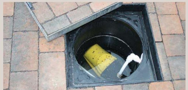
Around this home, rainwater runoff collected from all impermeable surfaces including roofs and paths, together with the 60m<sup>2</sup> permeable drive itself, passes into the tanked permeable pavement which contains a concealed sump. Here, a small pump is used to draw off the harvested water, in this case for outside uses, via a tap and hosepipe.
