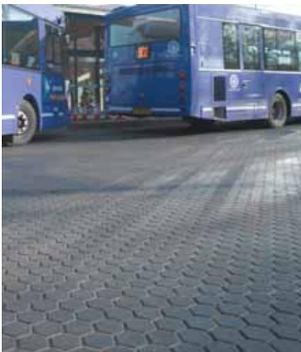
the constructed layers below and eventually into the subgrade. This effectively eliminates the requirement for additional drainage systems whilst also recharging the natural groundwater.
