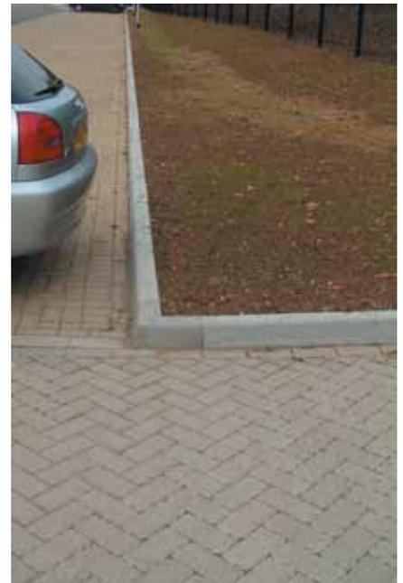
Under-drained, profiled verges are provided at the foot of banks and higher ground near permeable pavements to prevent silt and debris from being carried onto the pavement where blockage might occur.
