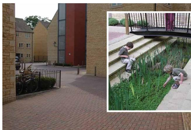
*Water controlled and cleaned by extensive permeable paving feeds directly into a planted canal, then to a river.*
