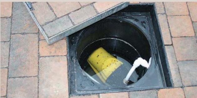
Around this home, rainwater runoff collected from all impermeable surfaces including roofs and paths, together with the 60m<sup>2</sup> permeable drive itself, passes into the tanked permeable pavement which contains a concealed sump. Here, a small pump is used to draw off the harvested water, in this case for outside uses, via a tap and hosepipe.
