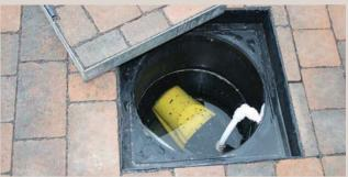
Around this home, rainwater runoff collected from all impermeable surfaces including roofs and paths, together with the 60m² permeable drive itself, passes into the tanked permeable pavement which contains a concealed sump. Here, a small pump is used to draw off the harvested water, in this case for outside uses, via a tap and hosepipe.
