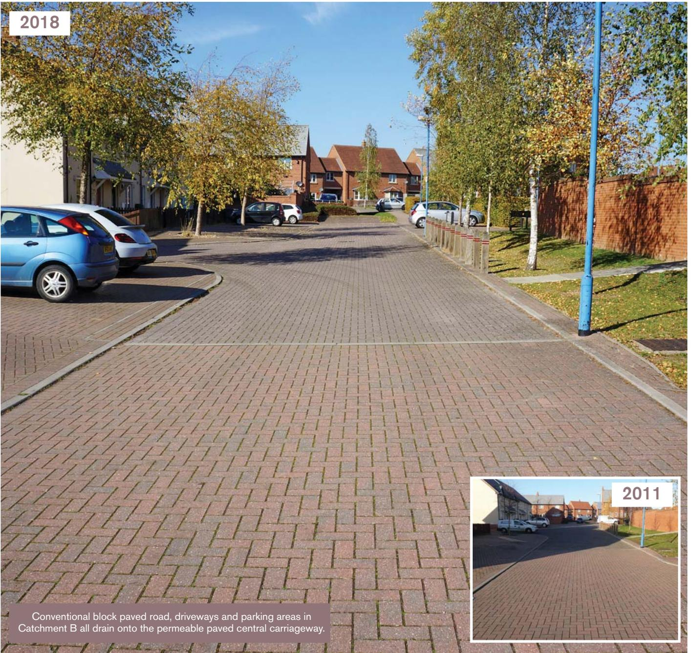
Conventional block paved road, driveways and parking areas in Catchment B all drain onto the permeable paved central carriageway.
