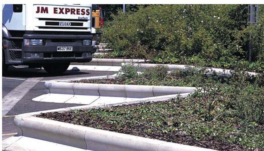
Precast concrete kerbs offer a complete range of components, whereas other materials with limited accessories may result in the need to mix different materials.
