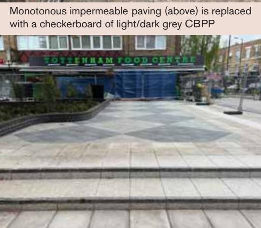
Monotonous impermeable paving (above) is replaced with a checkerboard of light/dark grey CBPP
