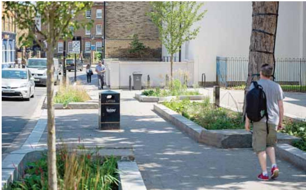
Permeable paving – using 600x300mm small-element concrete flags designed specifically for CBPP – was employed throughout pedestrian areas to the south side of the street facing shops, including the pocket park. It provides an attractive, safe and puddle-free accessible surface for all. In addition to providing a key SuDS feature, the CBPP between planters also provides a source of treated water and invaluable gas exchange (air in/CO<sub>2</sub> out) to the tree's root zone.
