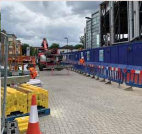
The CBPP paved highway withstood heavy construction traffic during the new station construction.
