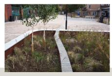
Australia Road, London - concrete block permeable paving laid over an existing road base collects rainwater and gradually discharges it horizontally into planted basins
