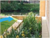
High-density housing in Stamford, Lincolnshire, where extensive concrete block permeable paving supplies planted canals with overflow directly to a river.
