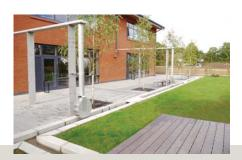
Bewdley School, Worcestershire - standard precast concrete units form rills handling rainwater from conventional concrete block paving and roofs – some via animated water features
