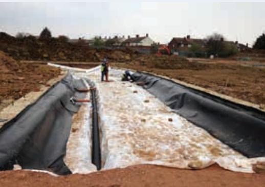
Central road base with drainage pipe in trench and inlets from driveways
