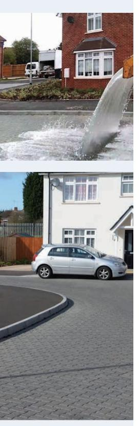
This case study demonstrates how concrete block permeable paved drives, parking and adopted roads can store and treat runoff from all the hard surfaces on a typical new housing development without any additional land-take or other SuDS features.
