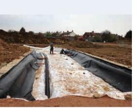
Central road base with drainage pipe in trench and inlets from driveways
