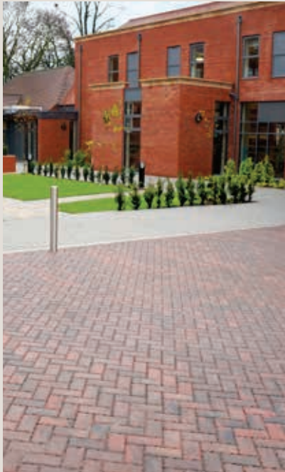
This low-level courtyard incorporates concrete flag permeable paving - which can be laid with or without spacers to achieve suitable joint spaces - as well as CBPP.
