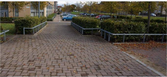
"Concrete block permeable paving is an ideal SuDS technique for high density housing, retaining a good quality finish with minimal maintenance."
