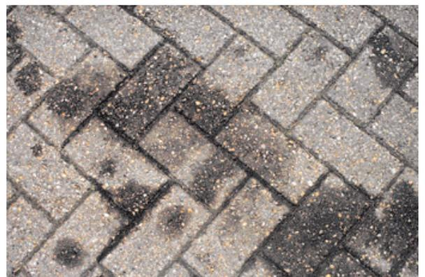
Alternatively the surface can be scrubbed with a strong detergent and the residue washed away with hot water. However, care must be taken as this method might also result in the leaching out of some pigment from the concrete product and discolouration due to surface abrasion of the concrete.
