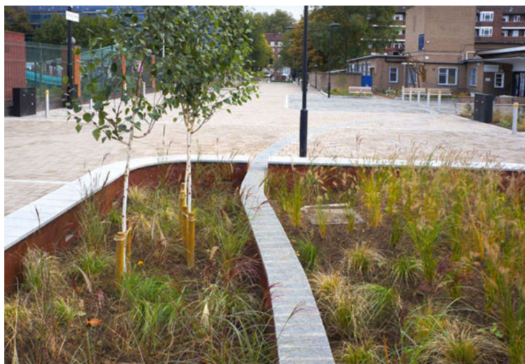
Figure 9: CBPP retrofitted over an existing road structure collects water and discharges it through slot drains into adjacent SuDS basins
