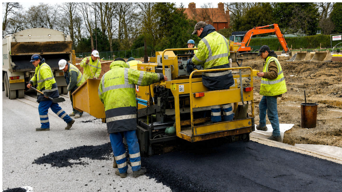
Figure 48: Tracked asphalt paving machine installing AC over a permeable sub-base
