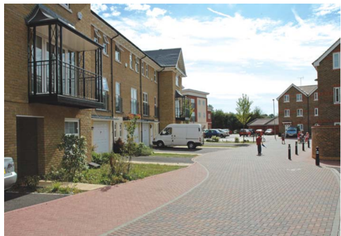
Figure 3: CBPP in a high density development.
