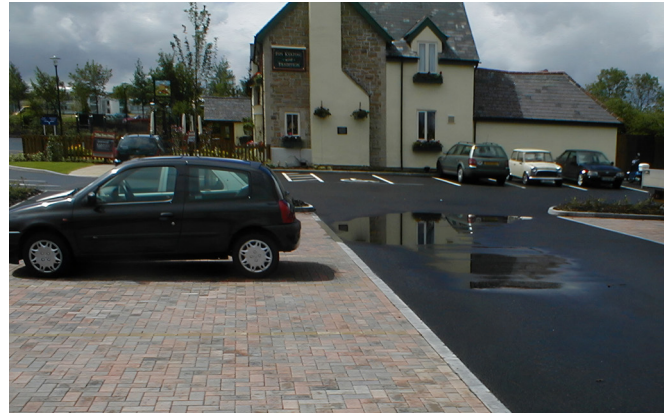
Figure 4: a demonstration of 'ponding' on impermeable asphalt paving, absent from adjacent CBPP under the same rain conditions.
