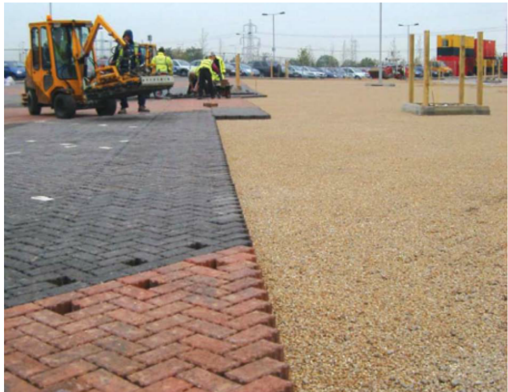
Figure 50: Machine laying of concrete paving blocks offers a particularly efficient solution for permeable as well as conventional block pavements
