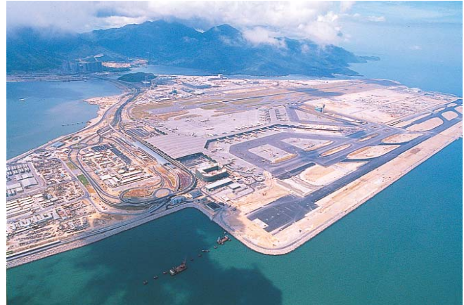
Figure 1. Hong Kong International Airport rests on native land and fill from two islands and soil dredged from the sea.
