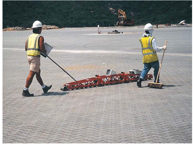
Figures 19 and 20. Checking surface tolerances with a straightedge and overall smoothness ensured a pavement amenable to keeping aircraft level during refueling.
