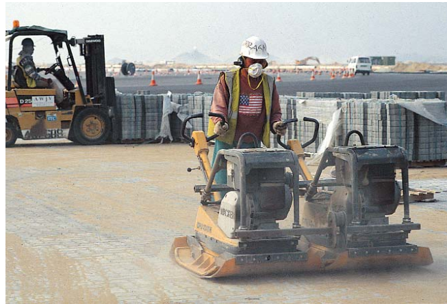
Figures 16 and 17. Dry joint was distributed across the compacted pavers and compacted into the joints until full. The joint sand gradation was finer than the bedding sand.
