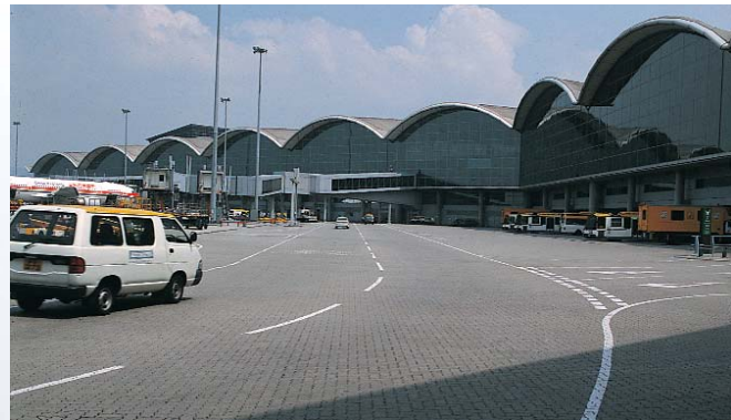
Figure 2. Interlocking concrete pavements were selected because they would tolerate expected settlement around the terminal building and remain serviceable.
