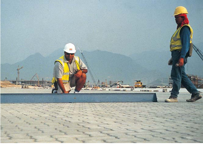
Figures 19 and 20. Checking surface tolerances with a straightedge and overall smoothness ensured a pavement amenable to keeping aircraft level during refueling.
