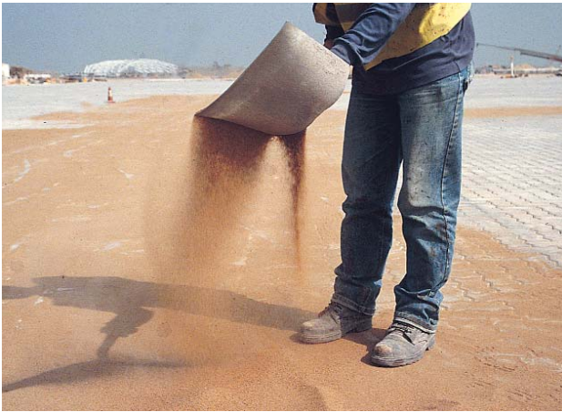
Figures 16 and 17. Dry joint was distributed across the compacted pavers and compacted into the joints until full. The joint sand gradation was finer than the bedding sand.
