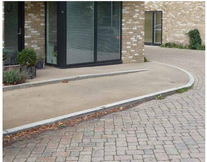
Precast concrete kerbs are used traditionally at road edges but also to form defined ramps for building access. 2011
