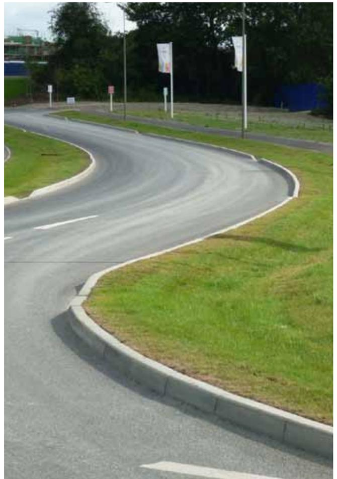
Enhanced swale with precast concrete dropped kerb inlets
