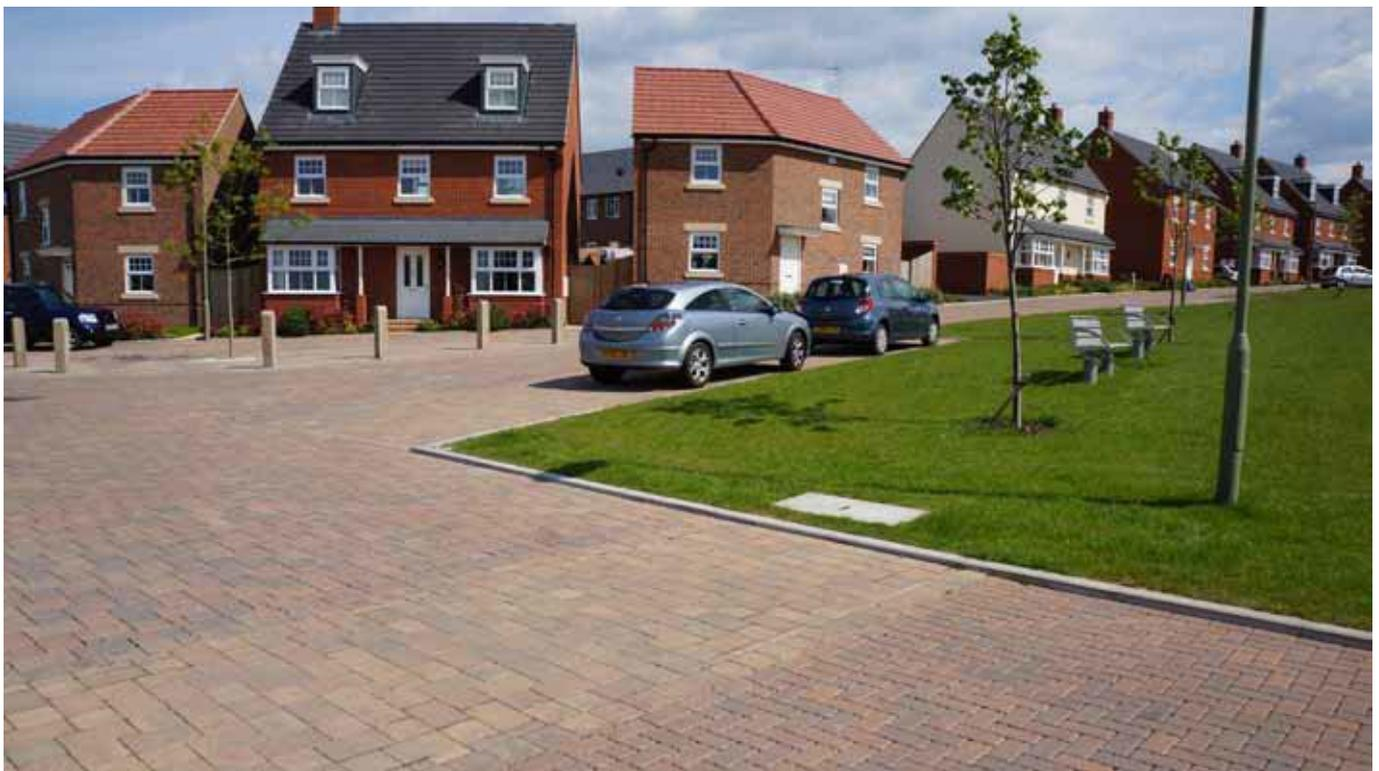
An impermeable paving service crossing within a permeable paved area
