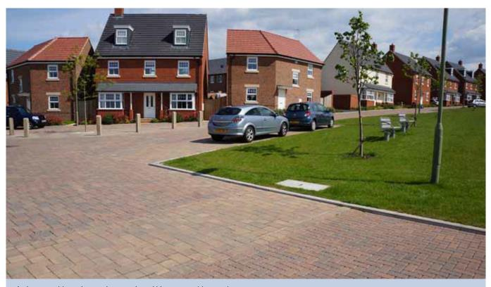
An impermeable paving service crossing within a permeable paved area
