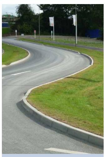
Enhanced swale with precast concrete dropped kerb inlets
