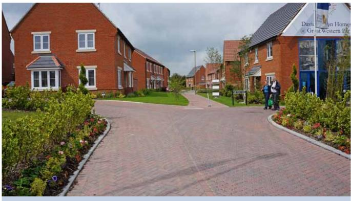
Permeable Paving drains adjacent impermeable surfaces as well
