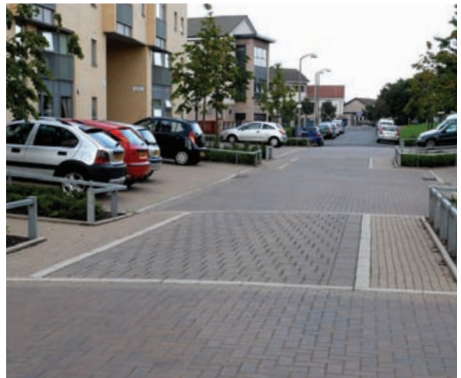
Concrete block permeable paving, combined with conventional block paving, is used throughout this major regeneration project in Craigmillar, Edinburgh.
