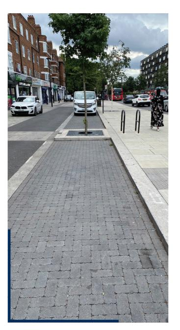
"CBPP works in synergy with trees, replicating natural permeable surfaces with diffuse rainwater infiltration and retention plus free air movement".
