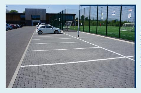
**Permeable Sub-base Extension** SuDS designers continue to innovate with CBPP, making the most of its capabilities to maximise performance and minimise costs. In the example shown left, the permeable sub-base of a car park extends below impermeable access roads and also an adjacent, artificial sports surface providing additional storage and adding to multifunctionality.
