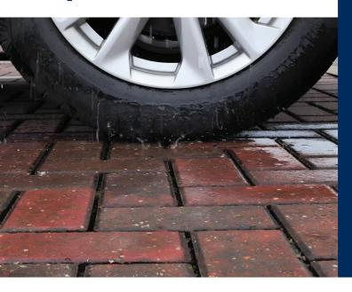
In contrast, rainwater drains straight off each block in CBPP, through the joints and laying course, as a permeable surface with dispersed drainage. CBPP attenuates and temporarily stores water during rainfall, cleaning, conveying and releasing it gradually over time. Essentially, it addresses flooding and water quality issues together, unlike attenuation tanks which only address flooding.
