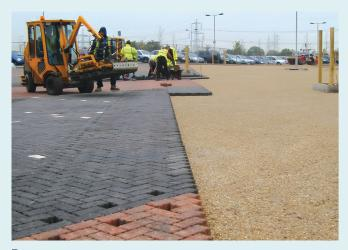
Machine laying of concrete paving units offers a particulary efficient solution for permeable as well as conventional block paving.
