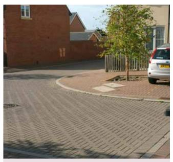
Concrete block permeable paving with conventional block-paved footways/ parking and flat kerb delineation.
