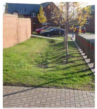
Under-drained swale B handles runoff from conventional block paving.
