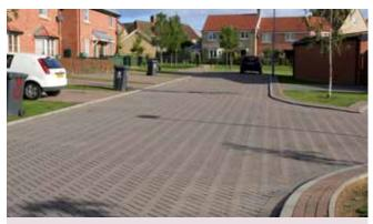
Concrete block permeable paved carriageway accepting runoff from conventional block paved drives and parking areas. Concrete kerbs laid flat delineate road edges.
