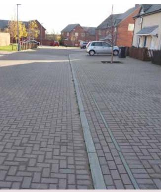
Precast concrete kerbs and various block laying patterns differentiate areas of paving.
