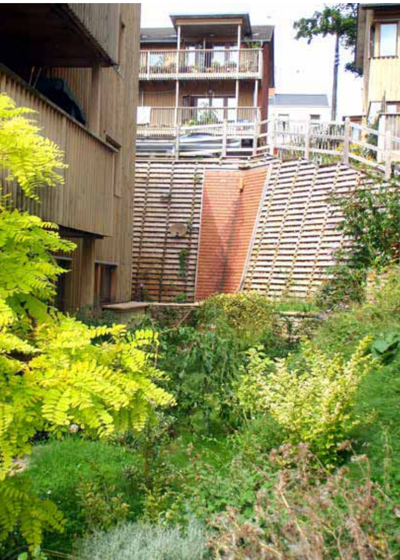
Spring Hill Co-housing, Stroud - concrete block permeable paving with flow control at the top of this hillside project discharges clean water to a cascade and planted swale, then a wildlife pond that also provides storage.
