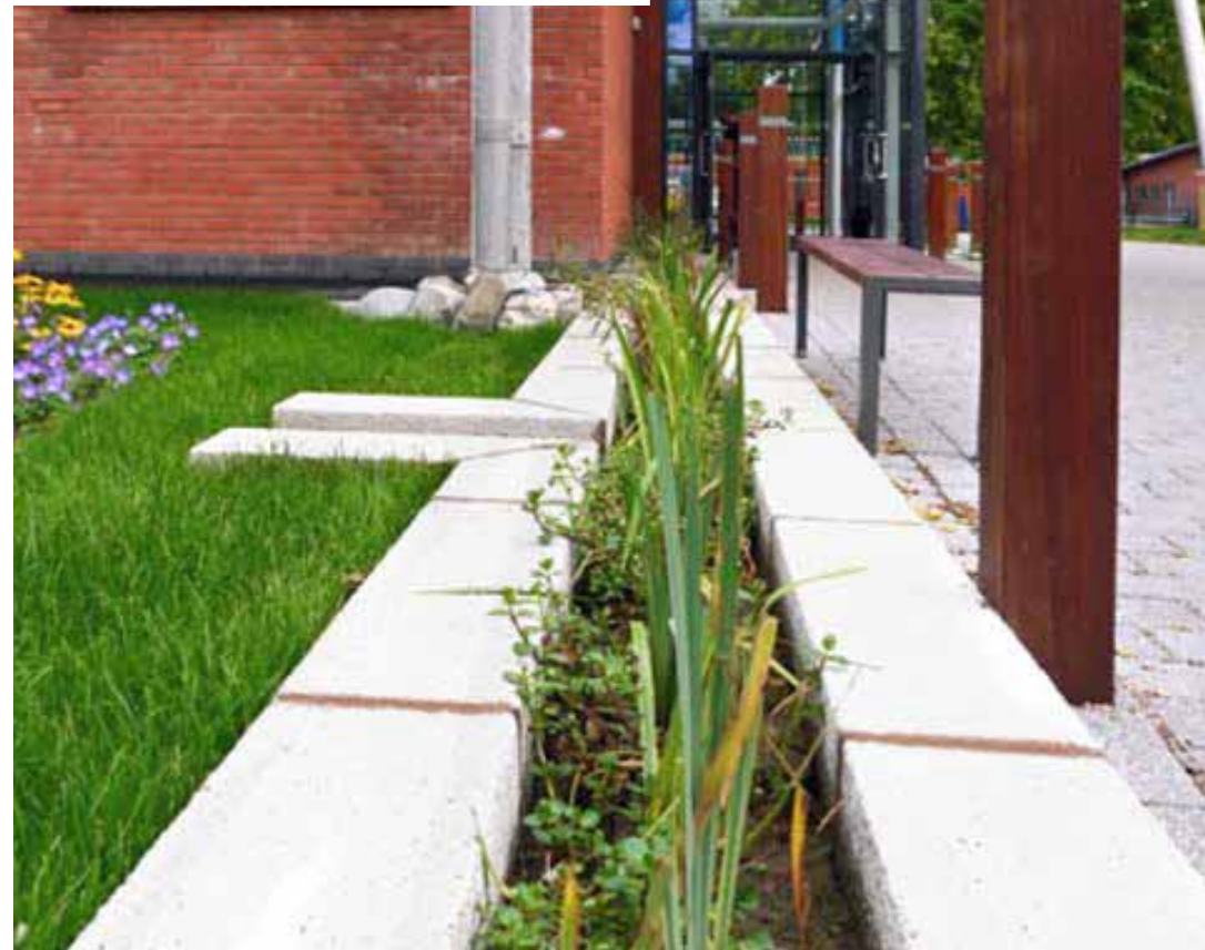
In the background, a downpipe discharges roof water through side perforations in changing patterns reflecting rainfall levels.
