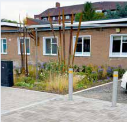
Sculptural metal rainwater elements feed into raingardens.
