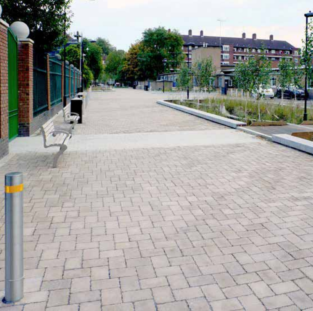
The original road surface has been replaced with attractive, 'self-draining' concrete block permeable paving.
