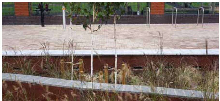
...to slots in side-walls discharging water from the permeable paving into planted basins.
