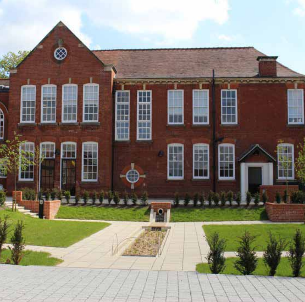
The main courtyard acts as a complete infiltration blanket with concrete block and flag permeable paving. The wetland rill is fed with roof water via a cascade, with some water stored and re-circulated by a solar-powered pump.
