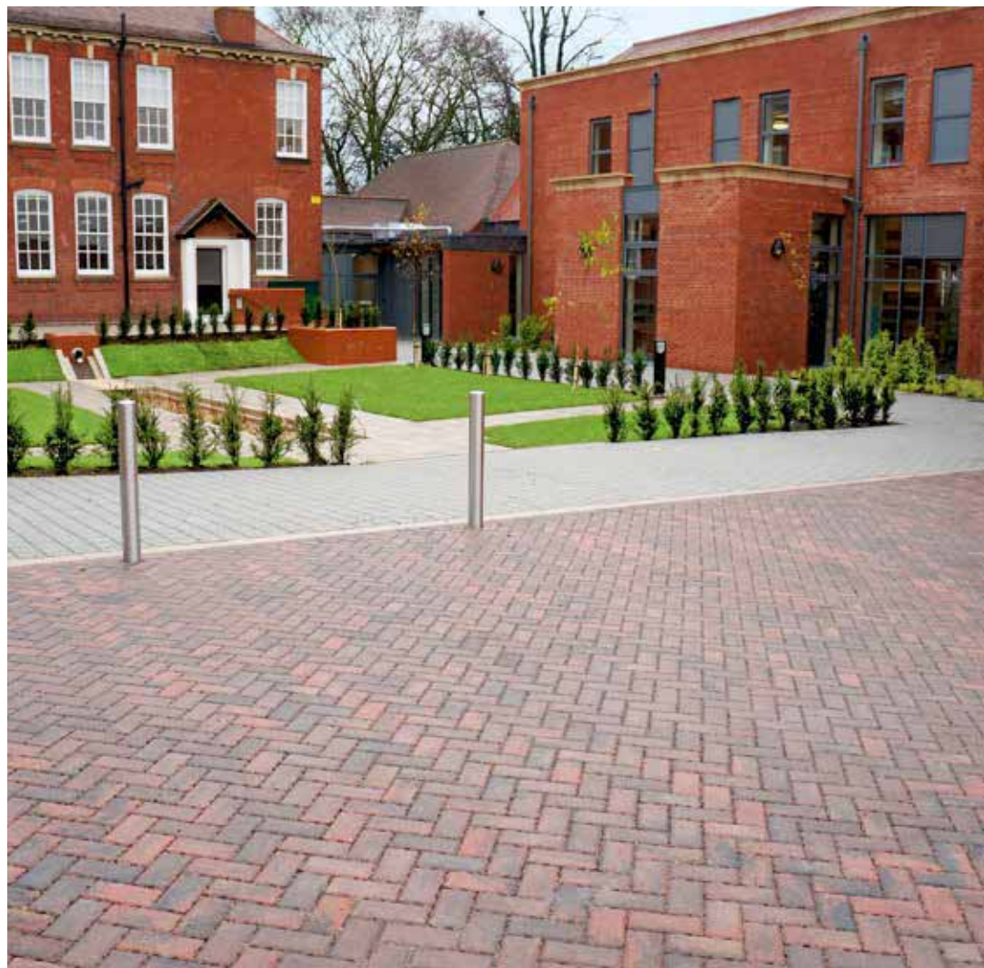
Parking areas adjacent to the courtyard are also concrete block permeable paving, differentiated by a red colour mix. The new library building to the right side completes the courtyard.
