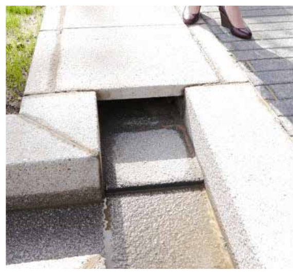
Standard precast concrete products are used in an interesting and attractive way to form rills.
