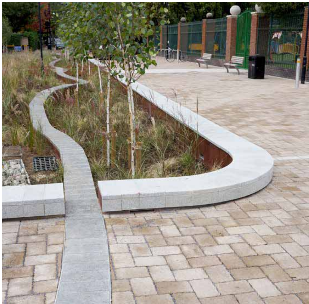
Clean water from the permeable paving passes into the planted basins. The 'wiggly wall' feature meanders through both paving and planting.
