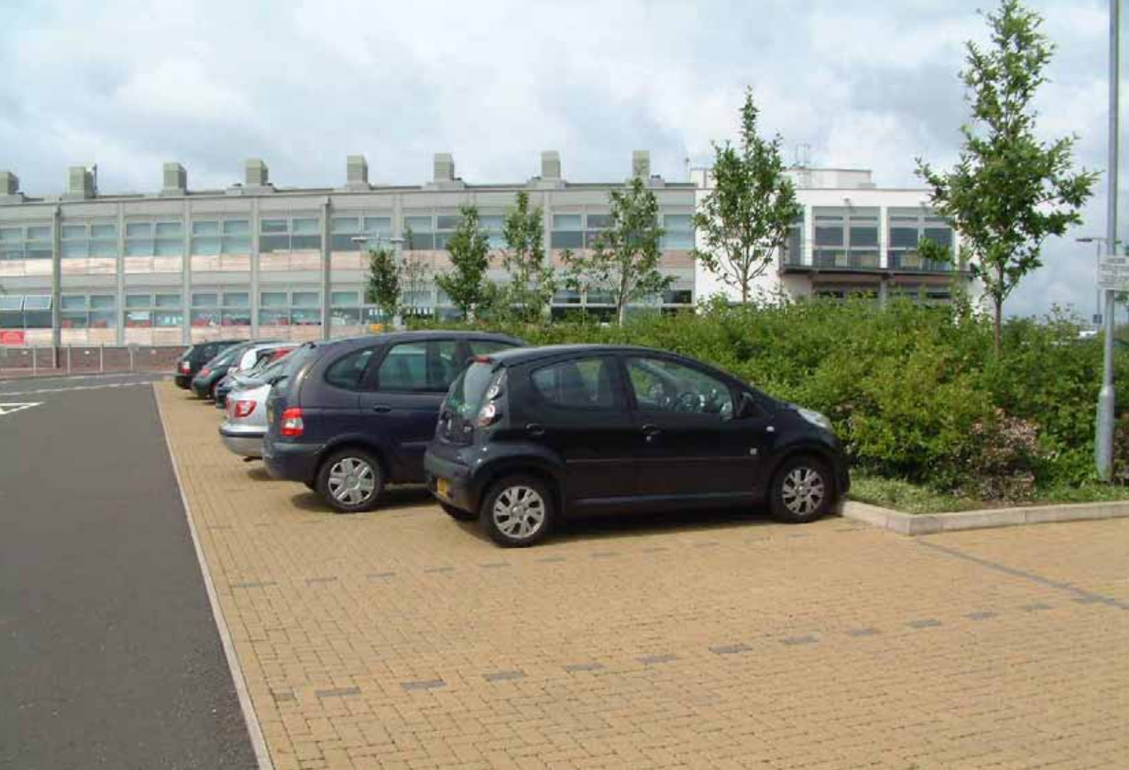
Hazeley Academy, Milton Keynes - designed on slopes, in terraced compartments with flow controls, the permeable paving supplies a steady flow of clean water to wildlife ponds inhabited by great crested newts.
