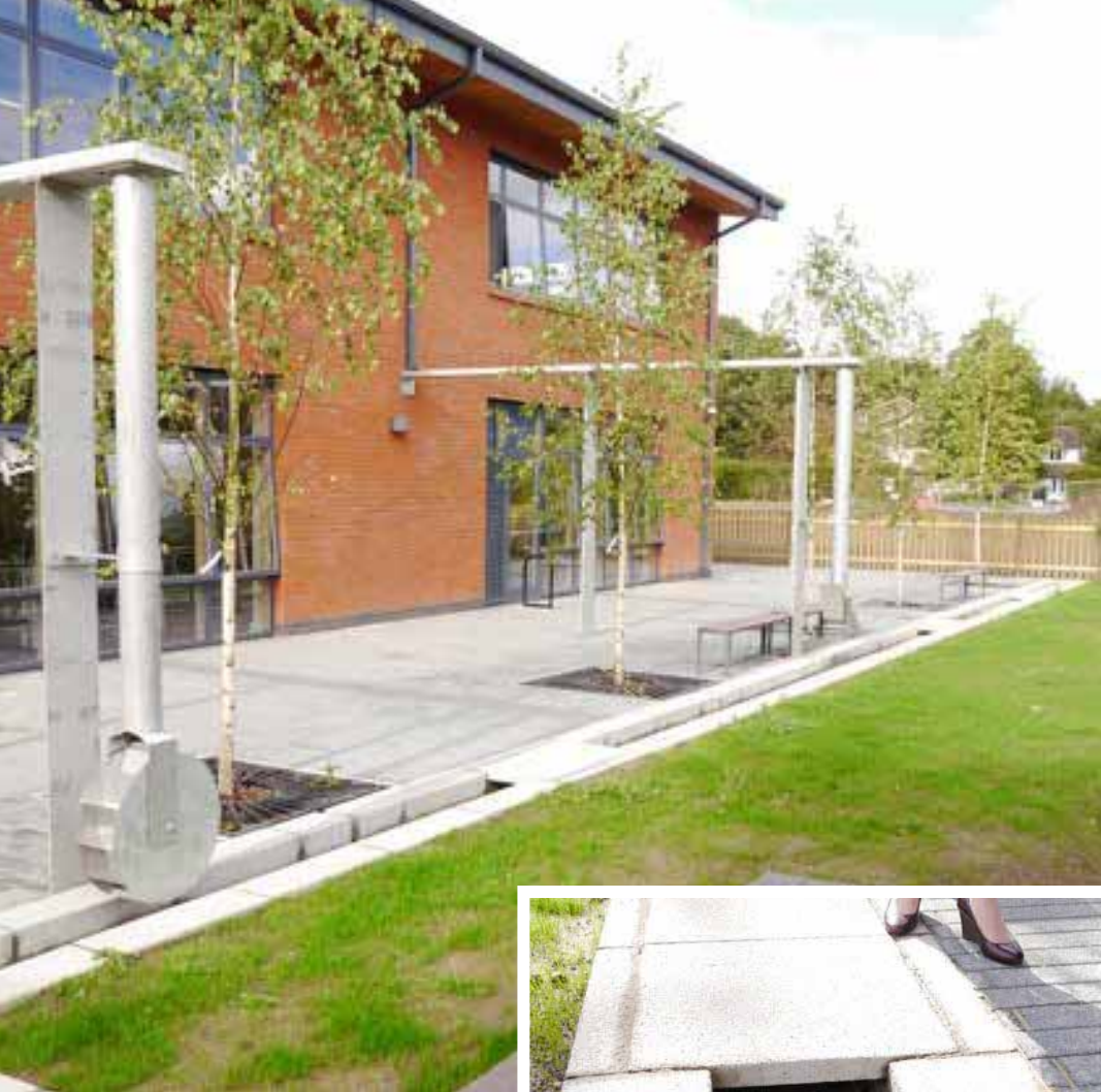
Standard precast concrete products are used in an interesting and attractive way to form rills.
