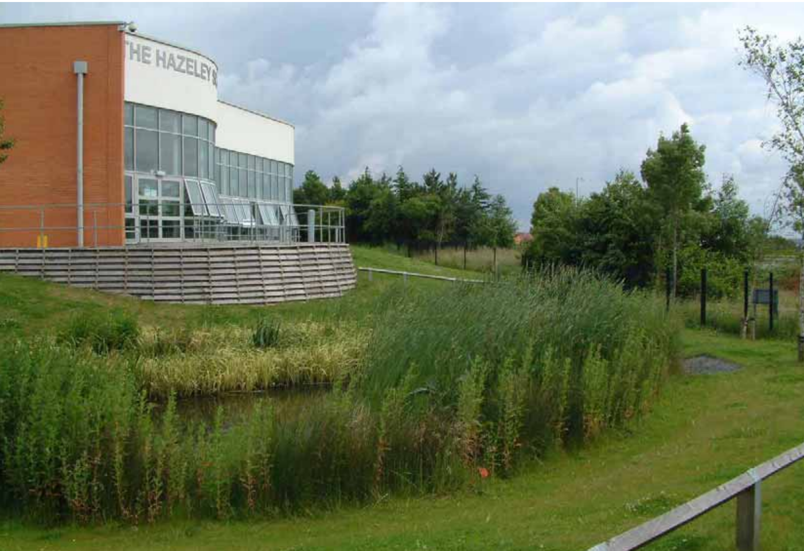
Hazeley Academy, Milton Keynes - designed on slopes, in terraced compartments with flow controls, the permeable paving supplies a steady flow of clean water to wildlife ponds inhabited by great crested newts.
