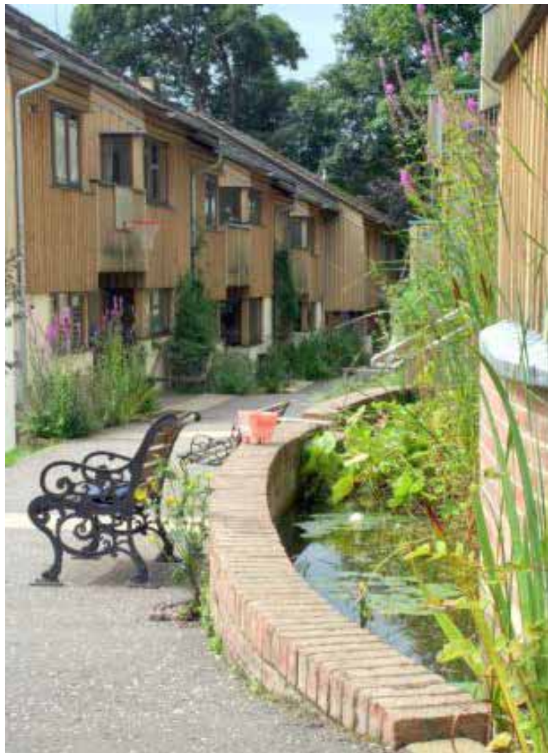
Spring Hill Co-housing, Stroud - concrete block permeable paving with flow control at the top of this hillside project discharges clean water to a cascade and planted swale, then a wildlife pond that also provides storage.
