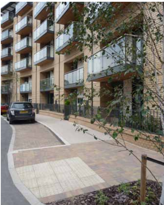
Realisation of the Design Code on a secondary road in an early phase with precast concrete paving
