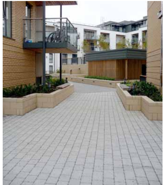
Concrete block permeable paving used for internal courtyards
