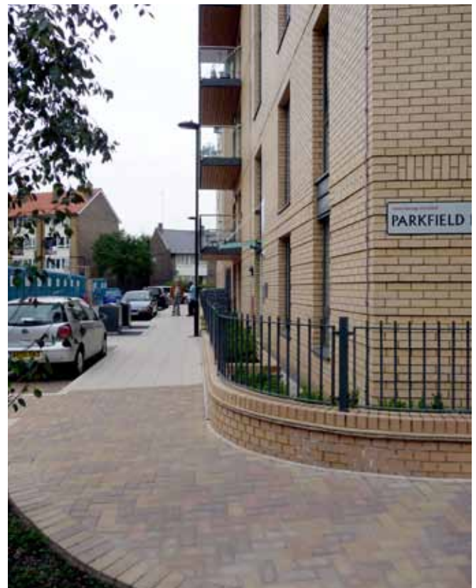
Concrete block permeable paving used for internal courtyards
