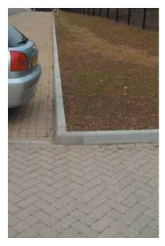
Under-drained, profiled verges are provided at the foot of banks and higher ground near permeable pavements to prevent silt and debris from being carried onto the pavement where blockage might occur.
