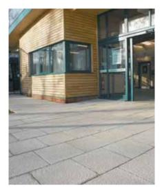
the constructed layers below and eventually into the subgrade. This effectively eliminates the requirement for additional drainage systems whilst also recharging the natural groundwater.
