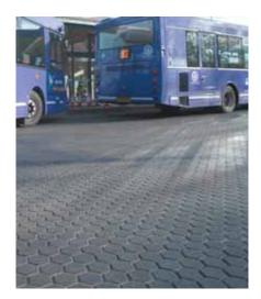
The project utilised 14,000 square metres of CBPP for circulation, parking and pedestrian areas, and local conditions allowed for a 'System A' form of construction with total infiltration of surface water to the ground. Here, all rainwater falling on the CBPP, and adjacent impervious areas draining onto it, infiltrates through jointing material,
