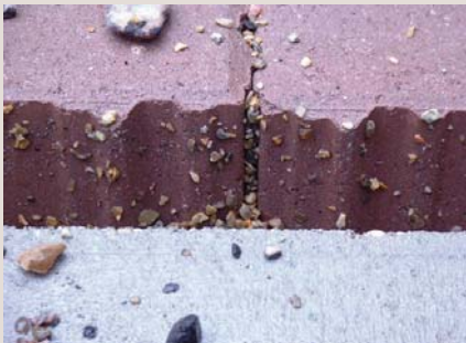
Figure 2: Principles of CBPP. As water passes through the pavement silt and other pollutants are also removed, which reduces downstream pollution.
