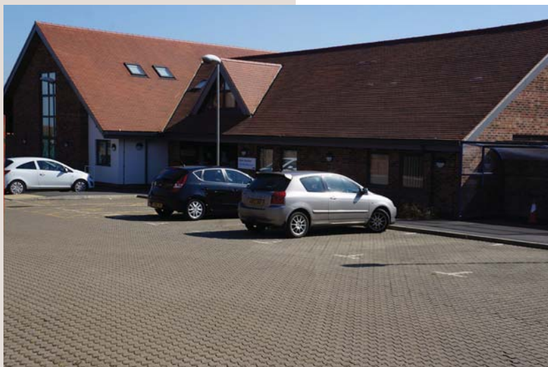
Figure 1: Example of CBPP at Upton Meadows Primary School, Northampton, in use since 2006.
