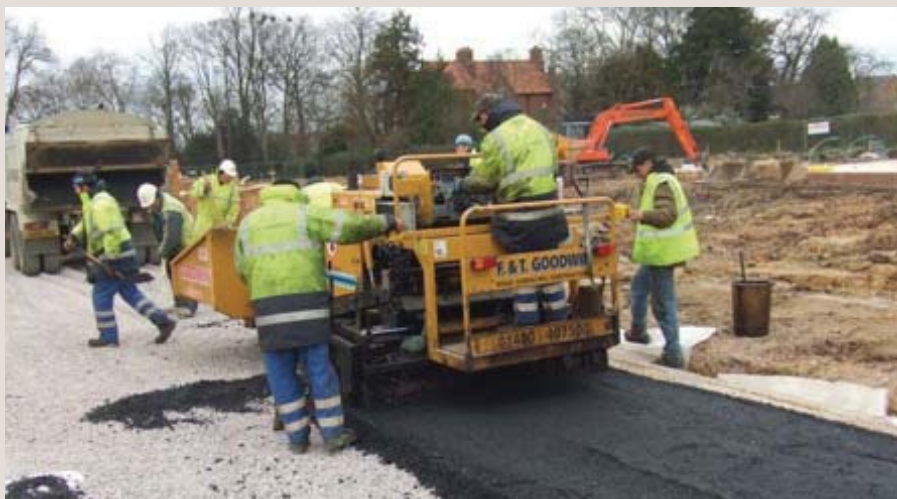
Figure 40: Tracked asphalt paving machine installing AC over a permeable sub-base.
