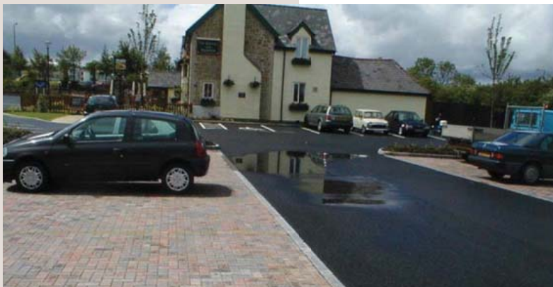
Figure 4: a demonstration of 'ponding' on impermeable asphalt paving, absent from adjacent CBPP under the same rain conditions.
