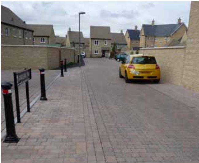
Pavements and crossing points at Carterton use impermeable paving for services, with visually matching permeable carriageways.
