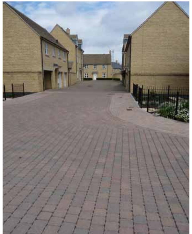
Later phases at Carterton use concrete block permeable paving.
