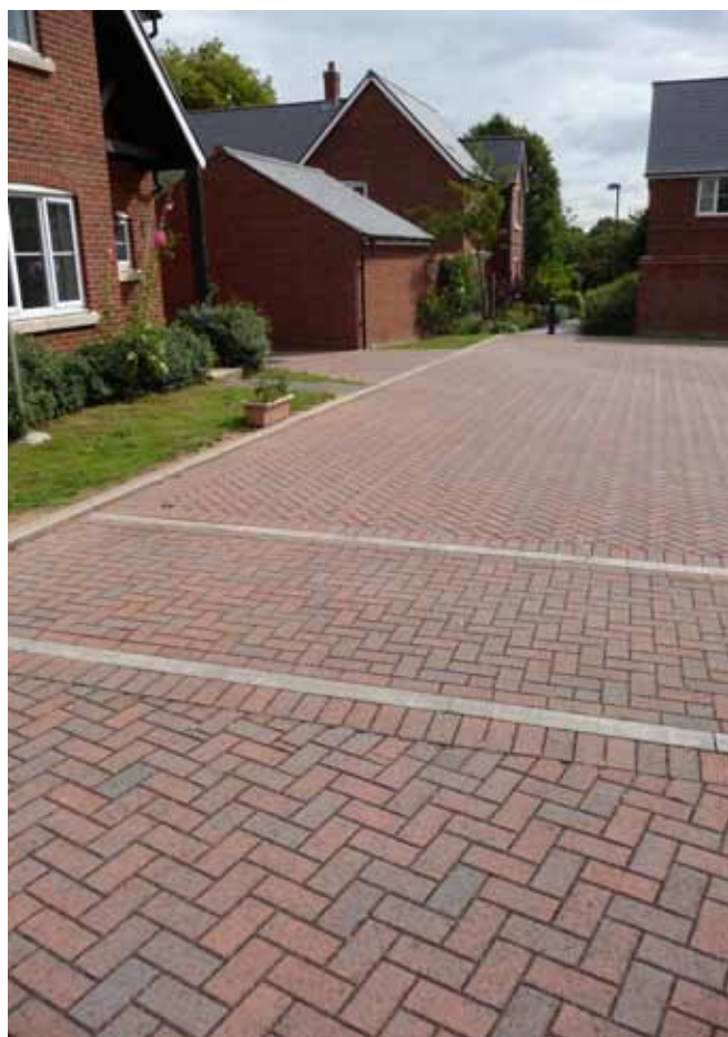
All services on this project - 'The Fairways', Kennington - run in verges or paving to the road sides then cross within distinctive impermeable block paving areas within the permeable pavement.
