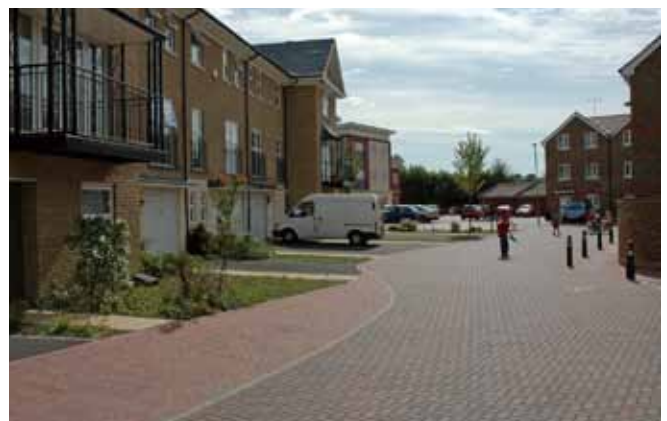
Saunders Road in Oxford is a large, new-build housing development built on the city's former bus depot site, over impermeable clay. It makes extensive use of concrete block permeable paving to treat and attenuate surface water runoff before gradual discharge to local sewers.
