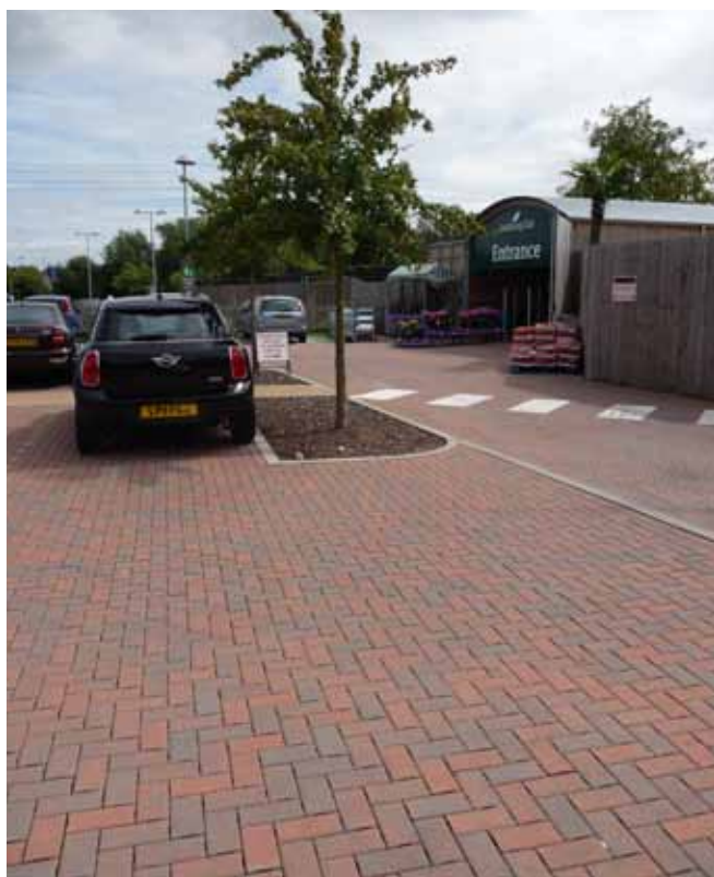
At Bicester Avenue Retail Park all the extensive car parking is permeable paving, at the head of the SUDS management train.
