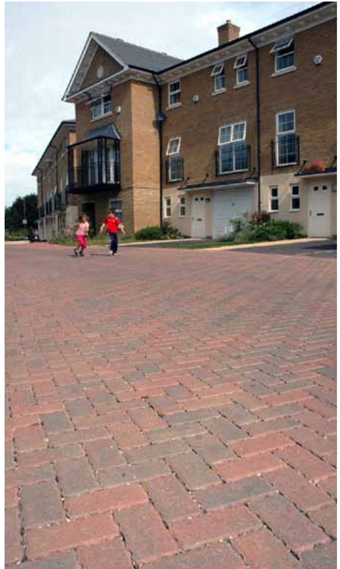
Saunders Road in Oxford is a large, new-build housing development built on the city's former bus depot site, over impermeable clay. It makes extensive use of concrete block permeable paving to treat and attenuate surface water runoff before gradual discharge to local sewers.
