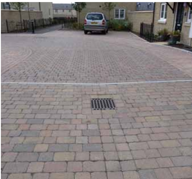
An earlier phase (foreground) at Carterton, conventionally paved with gulleys, has now been extended with concrete block permeable paving (background).
