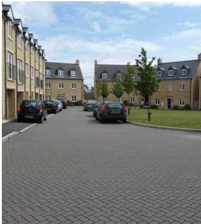
This project at Tower Hill, Witney, includes concrete block permeable paving within a conventional layout and used with raised footways and concrete kerbs which also retain soft landscaping.
