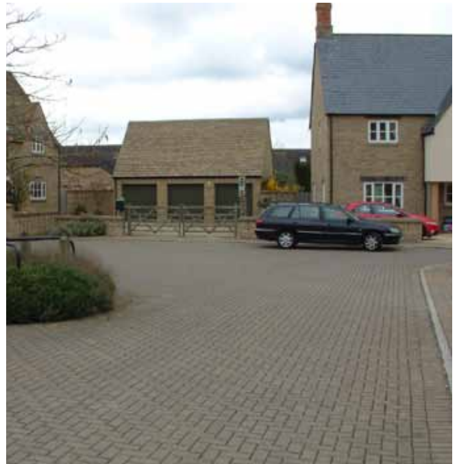
This modest scheme in the Thames-side village of Standlake has ground water just 18" below the paving surface and is immediately adjacent to the river and some lakes. During its 10-year life, the paving has been cleaned just once but it remains completely problem-free.
