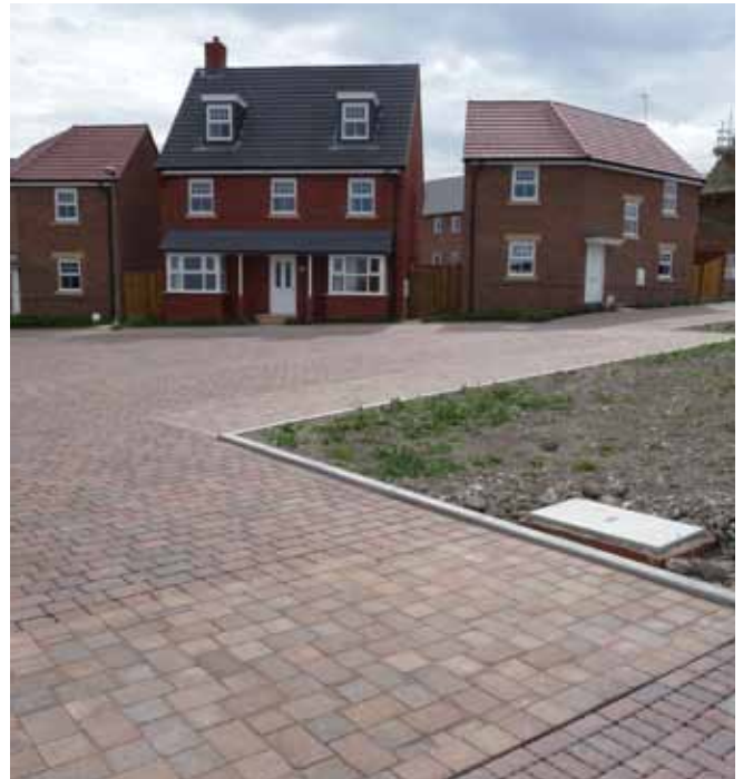
An impermeable service crossing through permeable paving under construction on the first phase of Didcot's Great Western Park.
