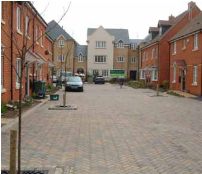
Wall-to-wall application of concrete block permeable paving with tree-pits provides sustainable drainage at this high-density development in Littlemore.
