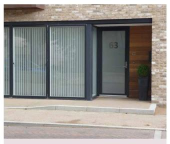
Concrete kerbs used to form a simple, consistent wheelchair access detail. 2011
