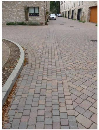
Tumbled concrete block paving in a single mix of colours is applied throughout with interest provided by use of pattern. 2011
