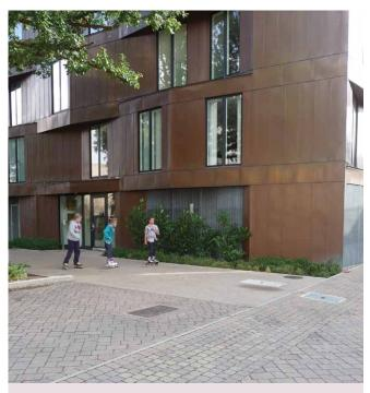
Varying block laying patterns and delineation with concrete kerbs and edgings defines different areas.  $\ 2011$
