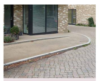
Precast concrete kerbs are used traditionally at road edges but also to form defined ramps for building access.  $\ 2011$
