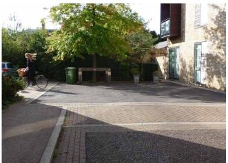
Raised 'Court' with block paved ramps and edges, highlighted by concrete kerbs laid flush. 2011
