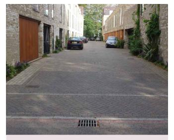
Concrete block paved transition zone with flush kerbs between mews and the main access road.  $\ 2011$
