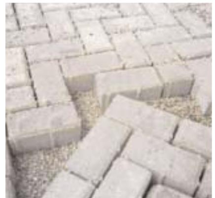
At Santos, rectangular paving blocks with oversize spacers were used as the surface to the permeable pavement.
