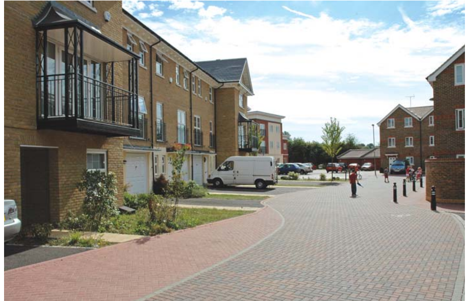
Figure 6: Concrete block permeable pavements in a high density development.
