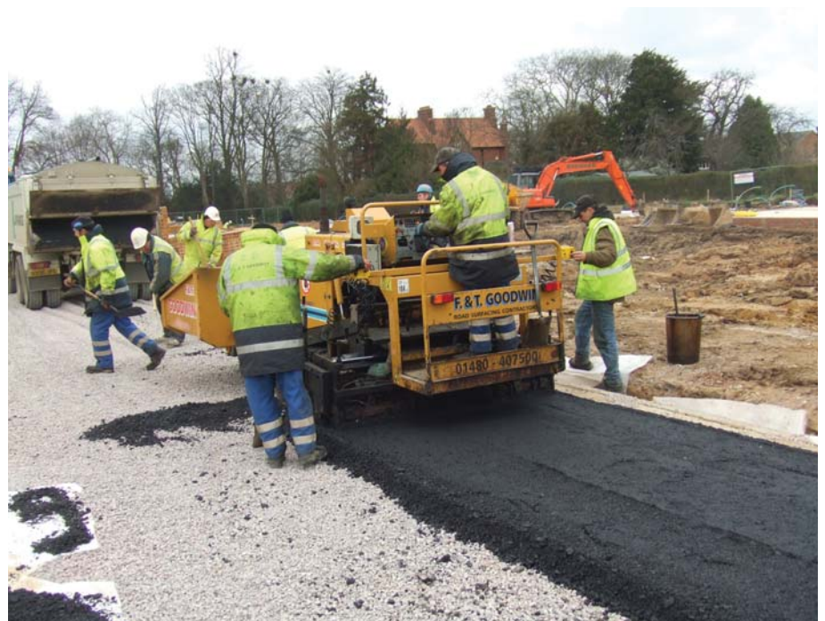
Figure 35: Tracked asphalt paving machine installing DBM over a permeable sub-base.
