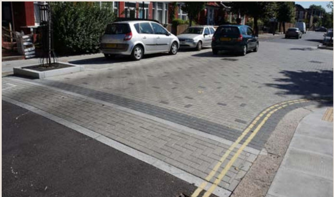
Precast concrete paving meets all these requirements and MfS highlights its own research demonstrating that block paving significantly reduces traffic speed compared with asphalt, particularly on shared surfaces. MfS2 also identifies a number of key characteristics, identified in ongoing research of shared spaces, where precast concrete paving can play an essential role, including:
