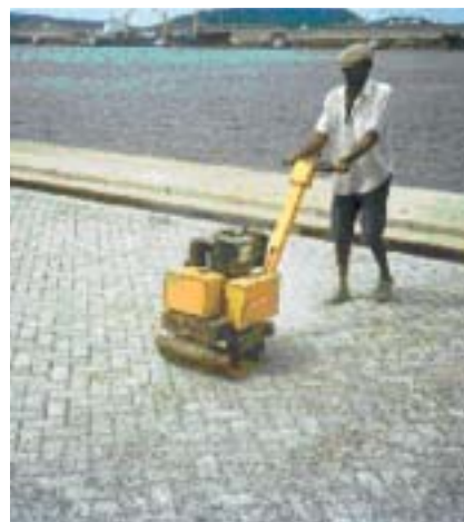
Completion of the permeable paving at Santos Container Port, Brazil.
