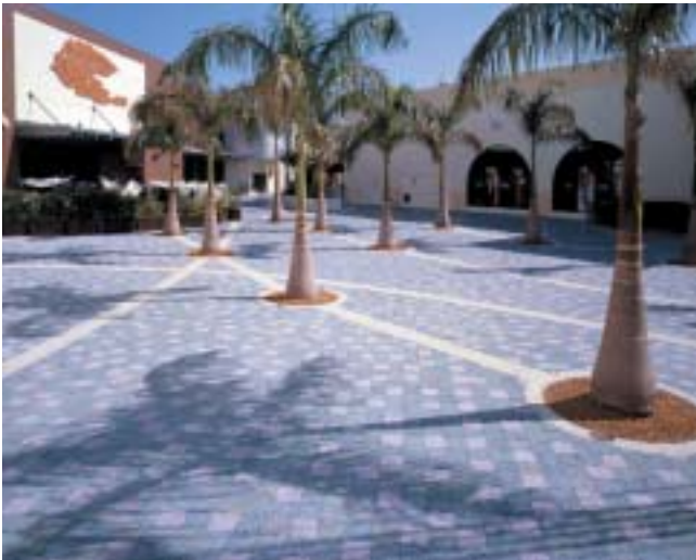
Surface treatment exposes glass and other special aggregates in the paving at this tribe-owned shopping centre in Hollywood, Florida (Honourable Mention).
