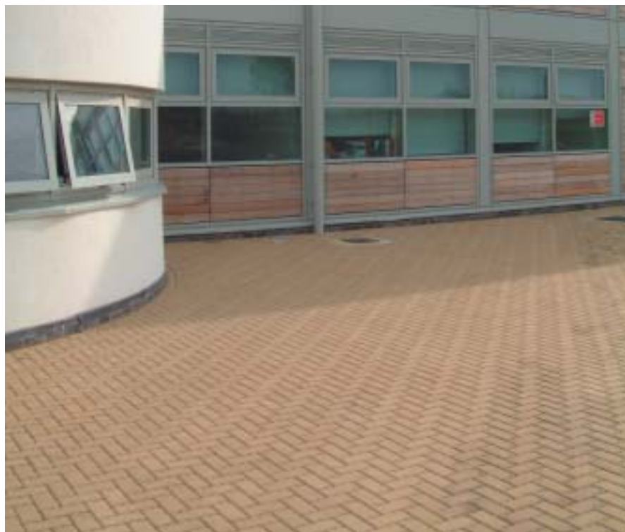
CBPP is used right up to the building at the Hazeley School and roof drainage discharges into the permeable pavement.
