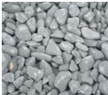
This sub-angular cement-treated roadbase was installed at a retail project in Dublin. Although the cement formed only a thin film layer coating the particles, it added significantly to the strength of the pavement.
