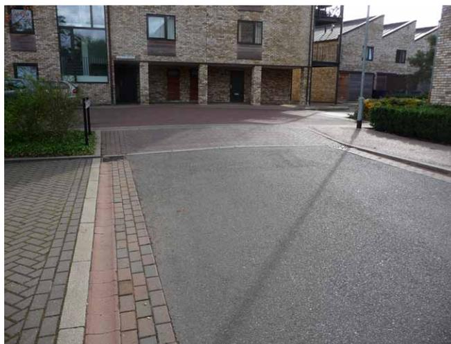
Charcoal, herringbone pattern block paving in car parks is contained by flush concrete kerbs with dished channels to gulleys. 2011
