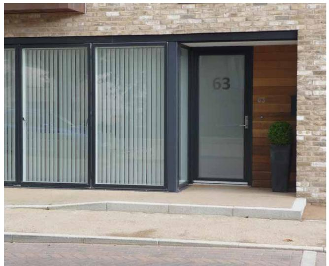
Concrete kerbs used to form a simple, consistent wheelchair access detail. 2011
